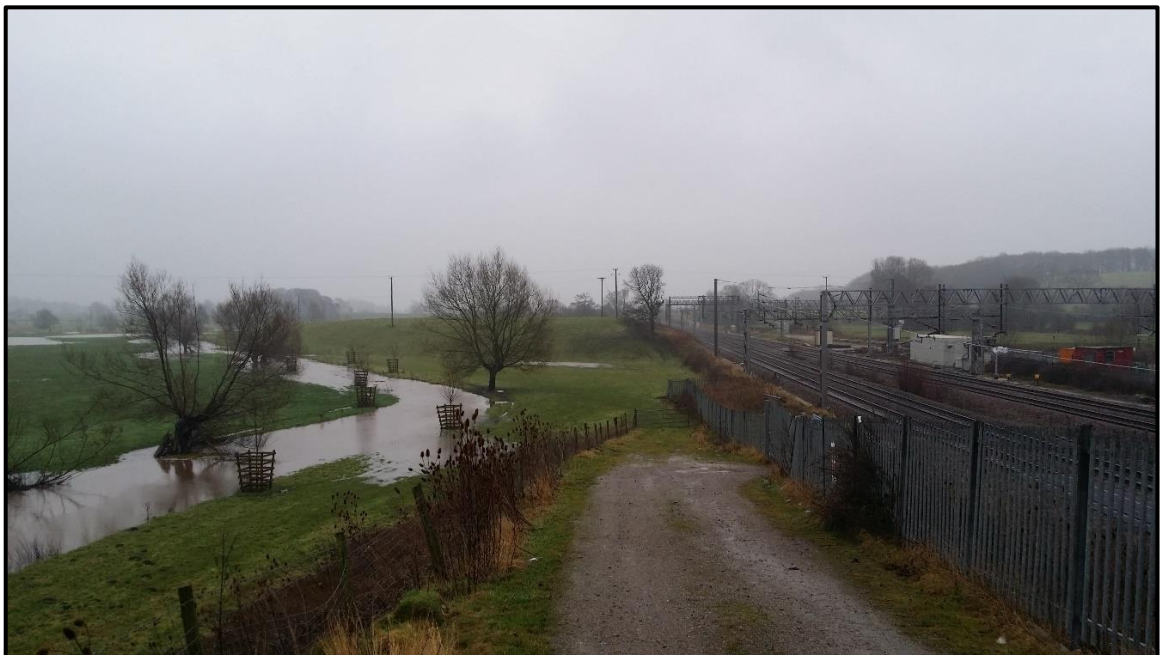
Figure 20 Flooding at Creswell, January 2017
