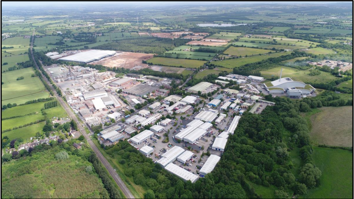
Figure 21 Aerial Photo viewing north east across the WMI site and surrounding industrial elements.
